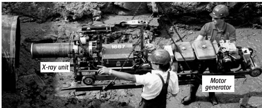
Fig. 12-18. Large diameter X-ray crawler with motor generator.
